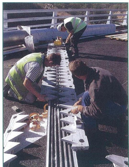
Assembly of aluminium elements and elastomeric profile outside the reservation
