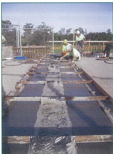
Drying of concrete before bolts tensioning
