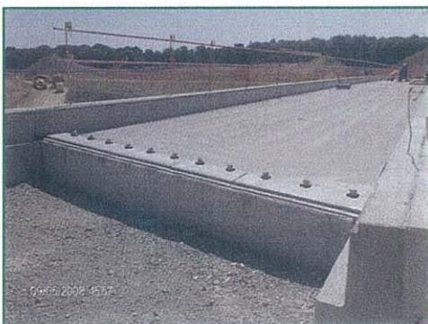
For railway bridges having a dilatable length less than 100 meters, ballast supporting joints are used.
