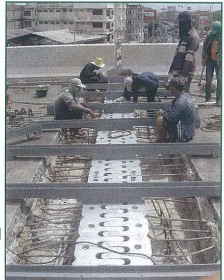
Malaysia / joint repairing – installation of a EJF400
