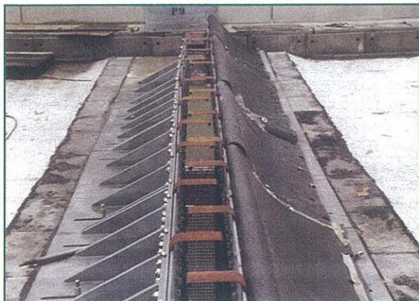
Each joint line follows the ballast cross section.
