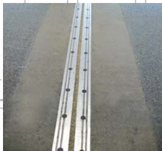
◆ Strip Seal Expansion Joint
