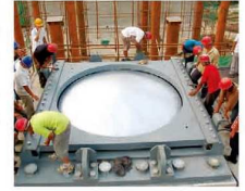
● The biggest tonnage bearing for highway in the world 160MN Spherical Bearing for Guangfu River Bridge, Jinming, Shandong Province, China
