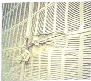
Picture of damaged soundproof wall
